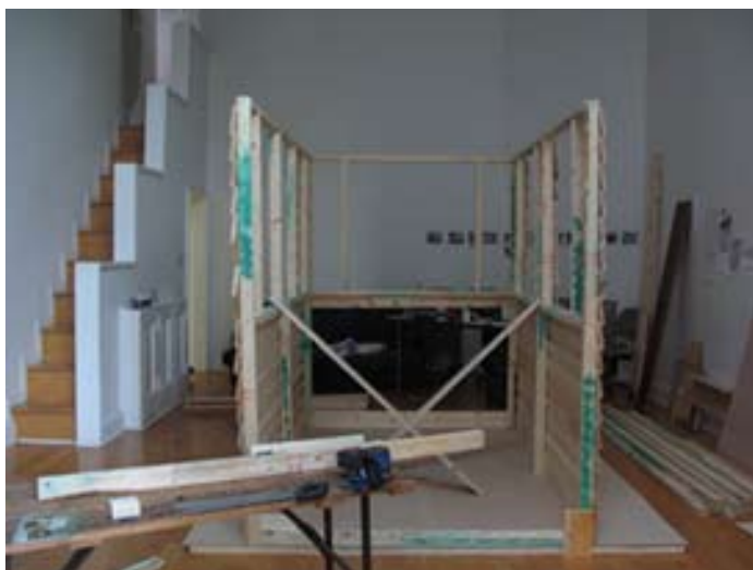
La construction solo
